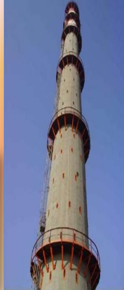
ARU/ SRU STACK
