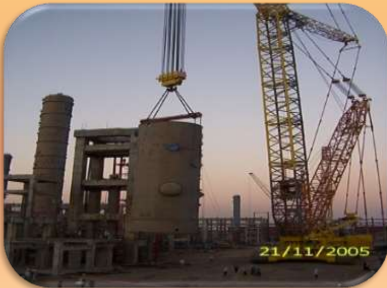
ERECTION OF 34RG-101 (REGENERATOR) = 298 MT DEMAG CC 12000
