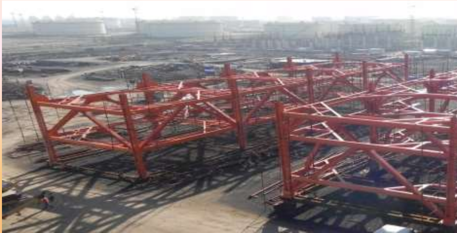
Coke drum structure module assembly
