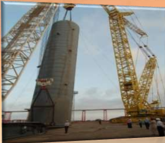
DHDS ERECTION – 960MT (DEMAG CC 12000 & CC 2500-1)
