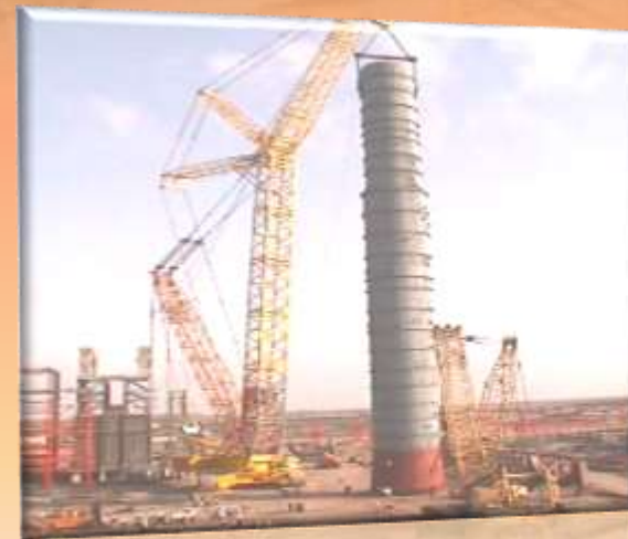
CRUDE COLUMN ERECTION – 685 MT (DEMAG CC 12000)
