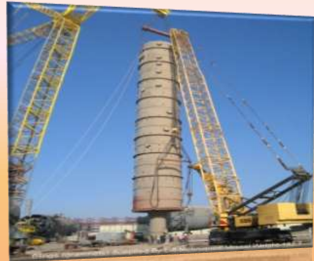
ERECTION OF 35C-101 – 182 MT DEMAG CC 12000
