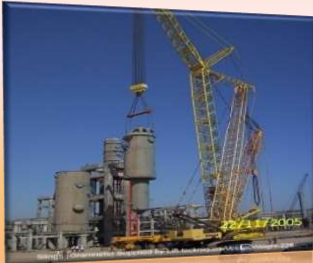
ERECTION OF 34R-101 – 225 MT (DEMAG CC 12000 & LR 1400)
