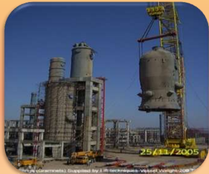
ERECTION OF 34RG-102 - 209 MT DEMAG CC 12000
