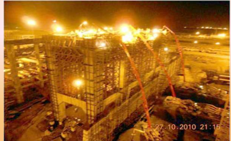
Deck slab casting
