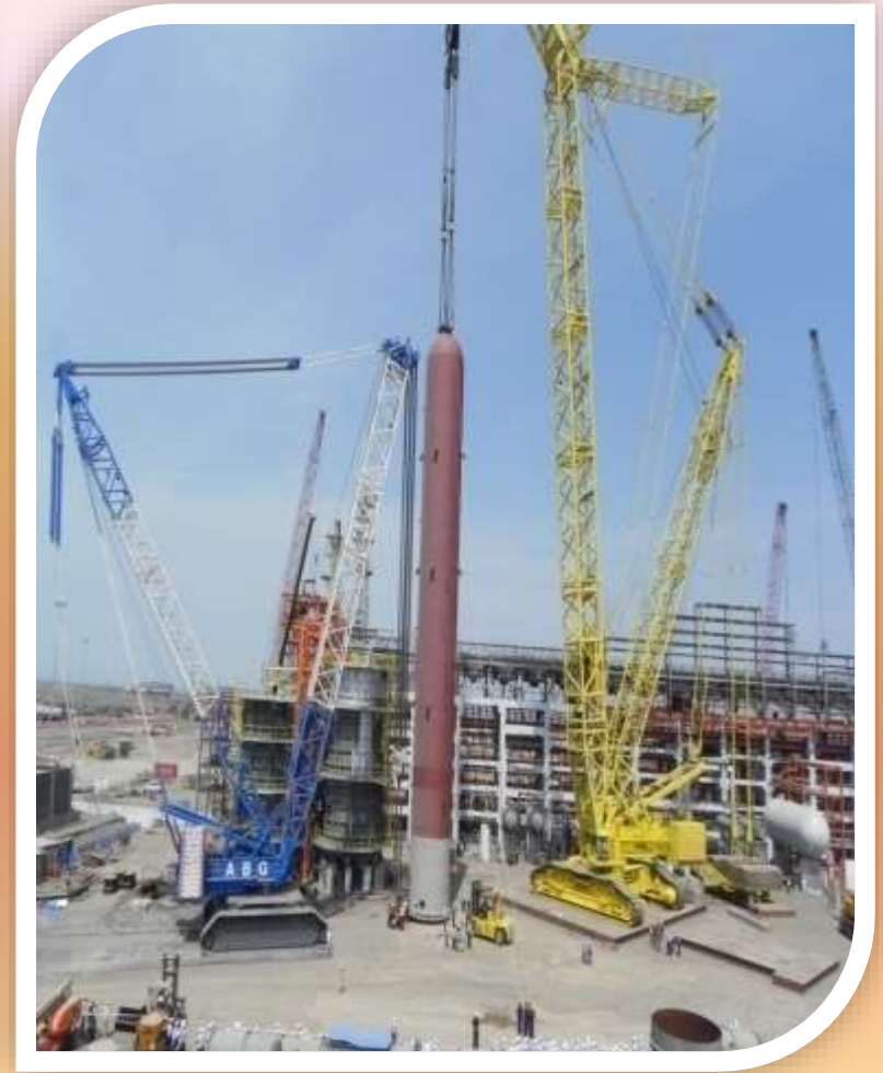
ERECTION OF DHDT REACTOR - 1300 MT - upgraded DEMAG CC 12000/SUPER LIFTER 1600
