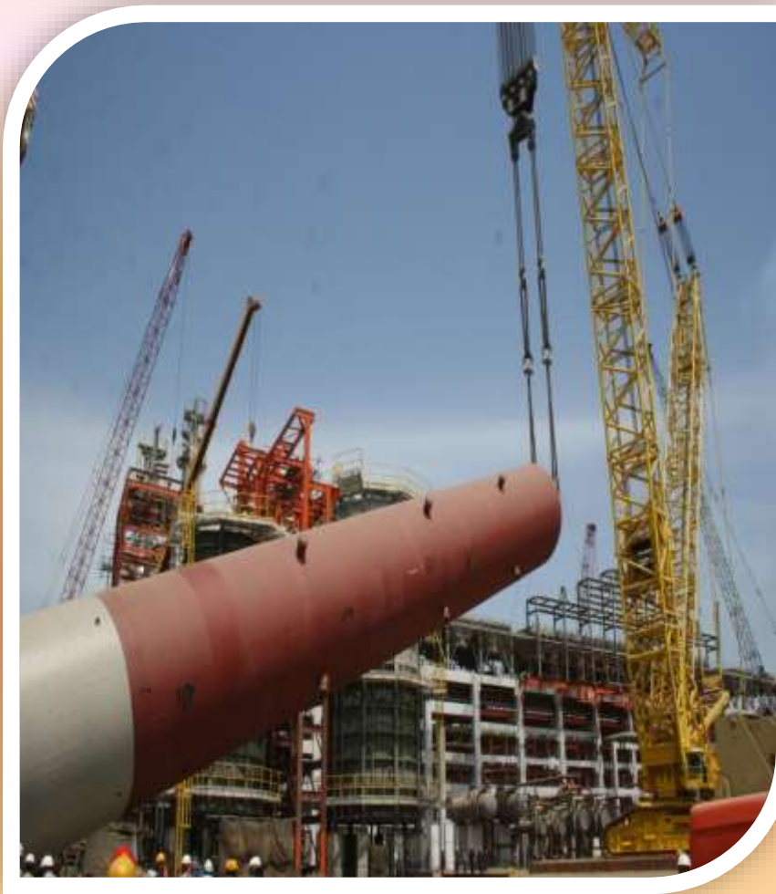
ERECTION OF DHDT REACTOR - 1300 MT - upgraded DEMAG CC 12000/SUPER LIFTER 1600
